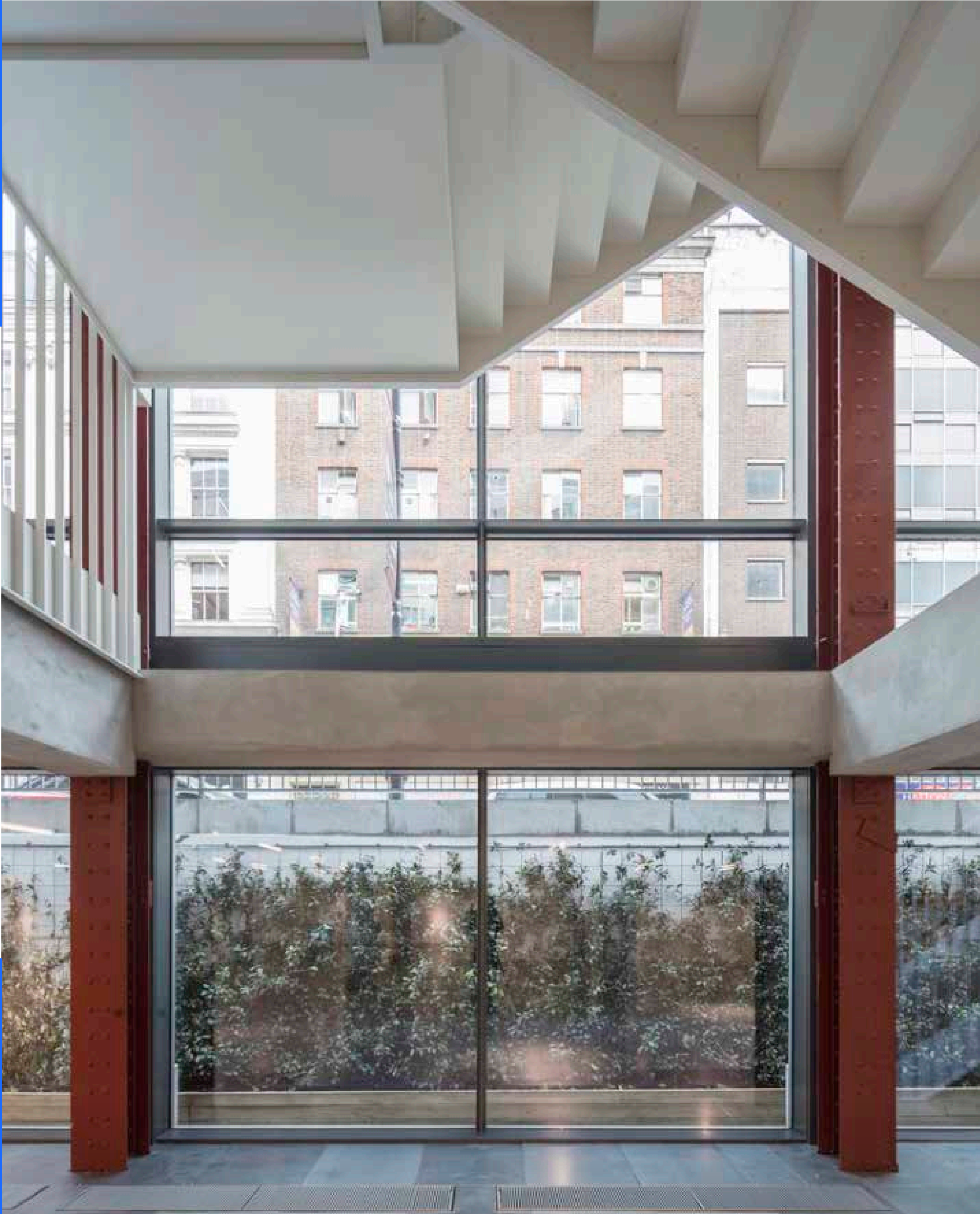
Lower ground floor glazed elevation (indicative photos)
